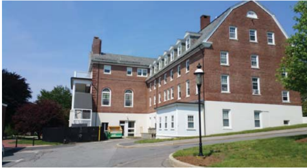
Camp Building View looking West
