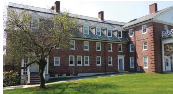
Camp Dormitory Wing Exterior
