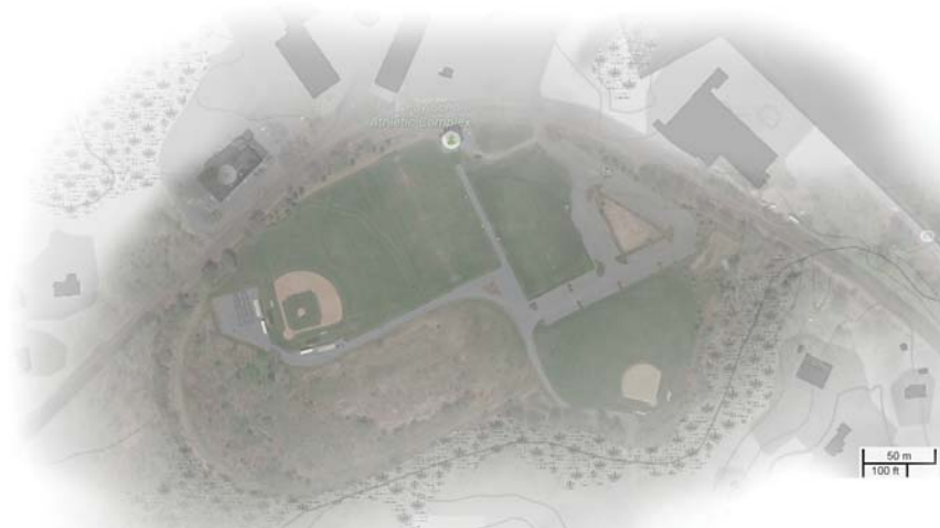
Existing Athletic Complex Aerial Photo
