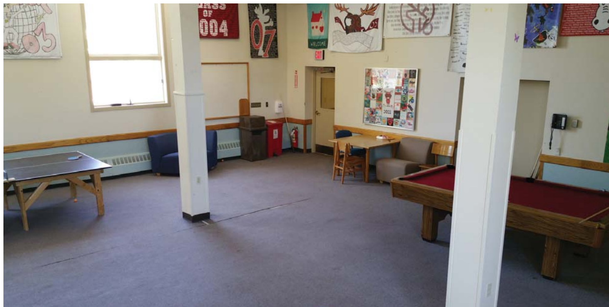
Camp Building - Existing Student Lounge
